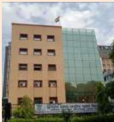
Installation of Tiranga at RC Building
